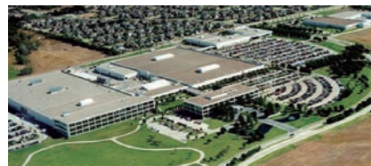
North America R&D Center (USA)
