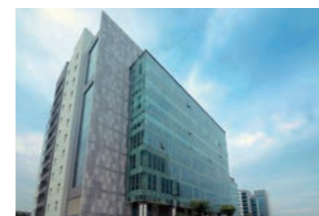
ABS Aircon Engineers Private Ltd. (India)
