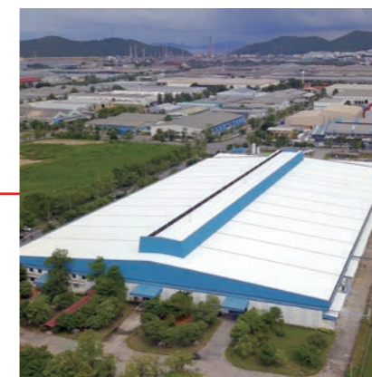
Fujitsu General (Thailand) Co., Ltd. (Thailand) Factory-2
